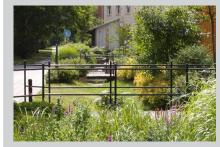
Linear vegetated features in which surface water can be stored or conveyed. Can be designed to allow infiltration where appropriate.
