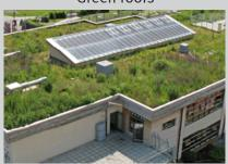
A multi-layered system that covers the roof of a building with vegetation/landscaping/permeable car parking, over a drainage layer. These features will not be considered for adoption by the SuDS Team.
