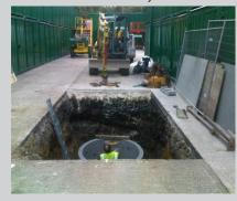
Square or circular excavations, filled with aggregate or lined with brickwork, or pre-cast storage structures surrounded by granular backfill.
