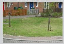
Surface storage basins that provide attenuation of stormwater runoff and facilitate settling of particulate pollutants. They are normally dry and may also function as a recreational facility.
