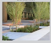
Shallow landscaped depressions or pre-cast units which rely on engineered soil and vegetation to remove pollution and reduce runoff.
