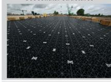
Modular geocellular systems with a high void ratio that can be used to create below ground infiltration (soakaway) or storage device.
