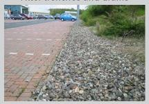
Shallow excavations filled with stone to create temporary surface water attenuation.
