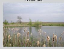
Shallow ponds and marshy areas for attenuation and water treatment. Aquatic vegetation and extended detention allow sediments to settle.
